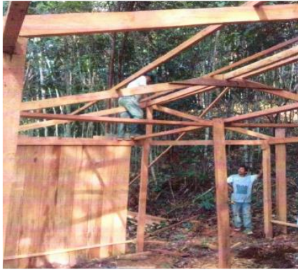
Illustration 9. Construction in Sector 3a
