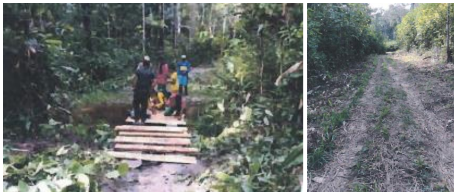
Illustration 27. Pedestrian bridge in Kirey Central and maintenance in road towards Corocito
